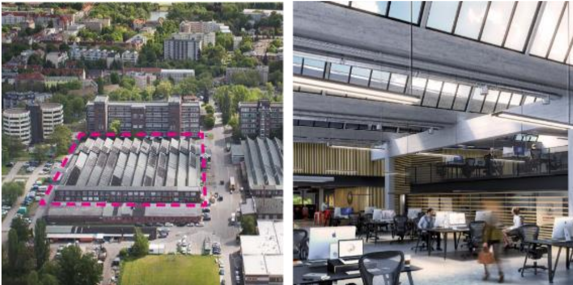
Figure 40. Innovation campus: (left) current status, (right) render of refurbished building
