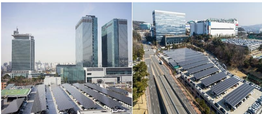
Figure 4.4 – Solar panels at parking lots in Samsung campuses in Korea [20]
